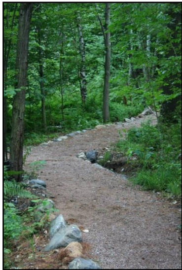
Stowe, VT - Stone Turnpike Cribbing
